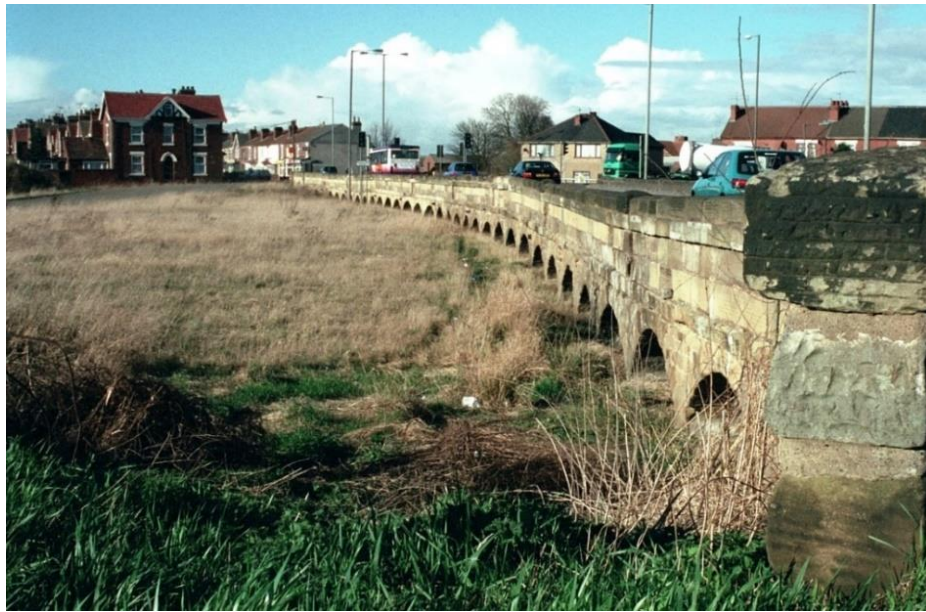
Fig.5. Bentley Causeway, known locally as “The Arches” (see map), was built by Doncaster-Selby Turnpike Trust in 1833. Many of the arches are original stonework but some have since been reinforced with iron plates and tie rods and a few renewed in brick. It was built following an 1832 Act “to provide safe passage over the River Don floodplain”. The whole area is only a few feet above sea level.
