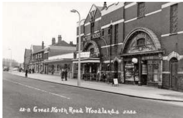
Woodlands: The corner of Princess Street and the Great North Road.
